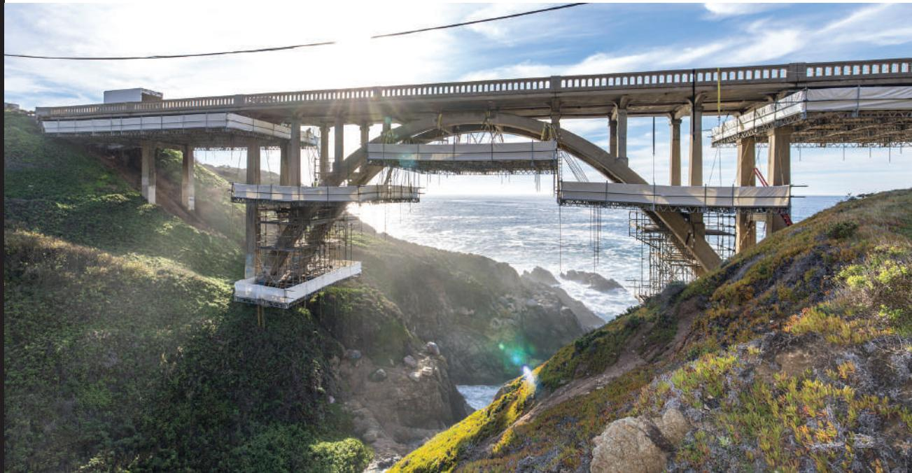
BrandSafway (**No. 4**) designed several multi-tiered suspended work platforms for use on the rehabilitation of the 90-year-old Granite Canyon Bridge in Monterey County, Calif. The 288-ft-long structure required a no-drill access solution that the firm says would not jeopardize the integrity of the center span or interfere with the bridge's anti-corrosion system.
