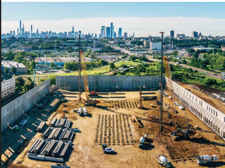
As part of the Lincoln Gateway project, Menard Group USA (**No. 166**) installed rigid inclusions to depths of up to 175 ft to support a 326,000-sq-ft distribution center in Secaucus, N.J., the firm says.
