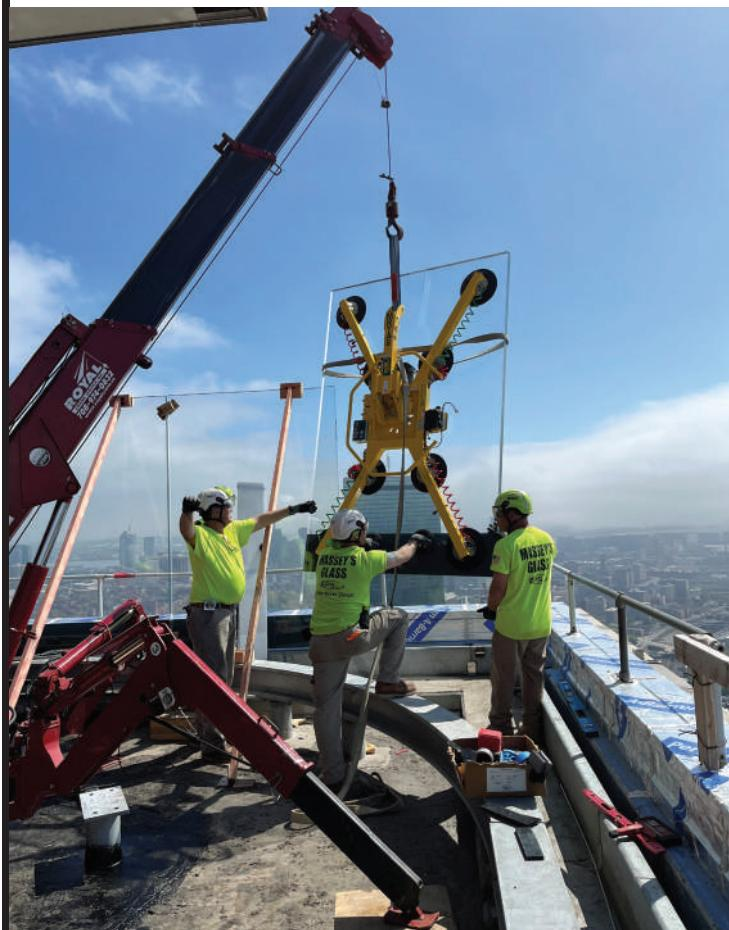
Massey's Plate Glass & Aluminum Inc. (**No. 273**) installed a 10-ft-high glass observatory around the perimeter of the roof deck at Boston's Prudential Center. All materials, including equipment and 3-in.-thick glass panels, were lifted to the 56th floor by derrick crane—with each lift taking 45 minutes.
